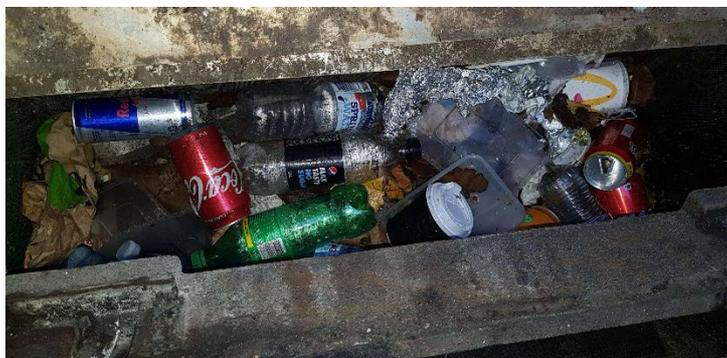
Image 1: Litter captured in an at-source litter trap installed in a stormwater drain
